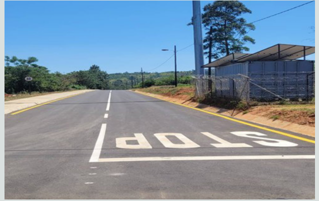
Completed Titandini Road
