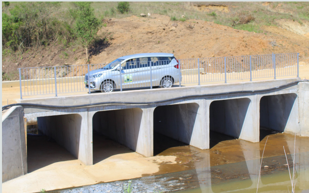
Completed D2 Bridge
