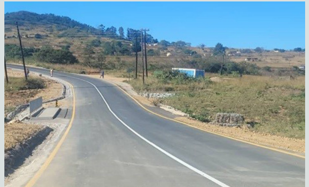
Completed D2 Bridge and Section of D2 Road
